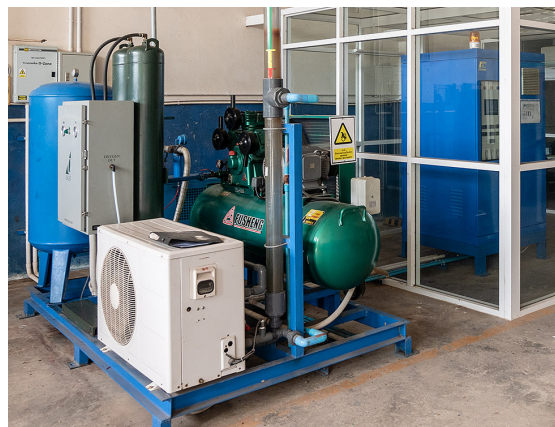
Ozone generating system at fishmeal plant in Thailand
